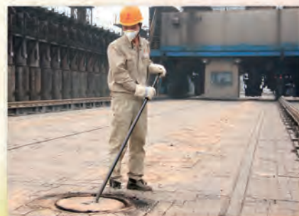
●炉盖工松动炉盖
